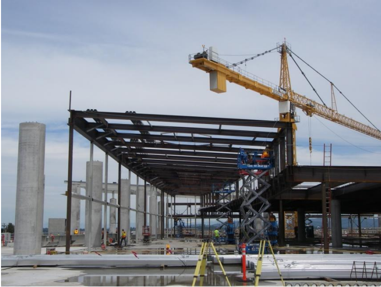
Customer Service Building & High Roof Progress
