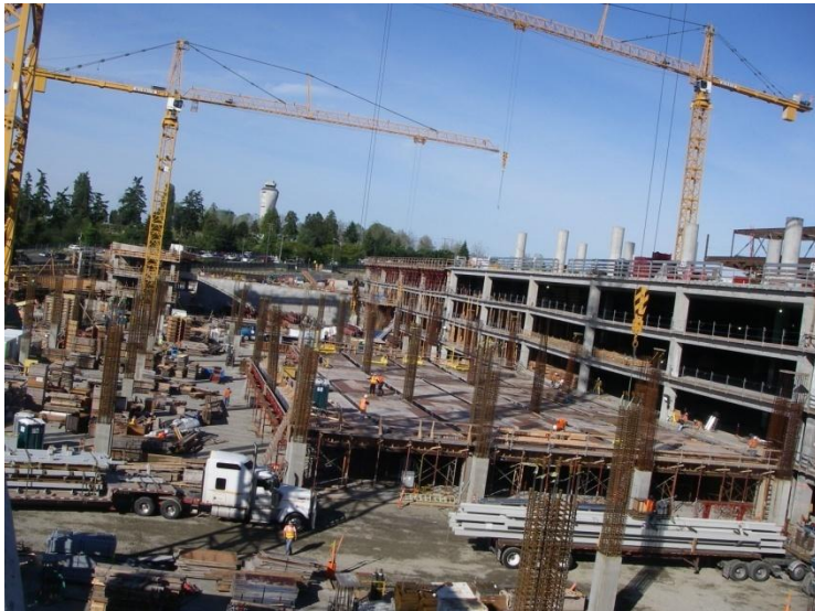
RCF Building Area E Elevated Deck Forms
